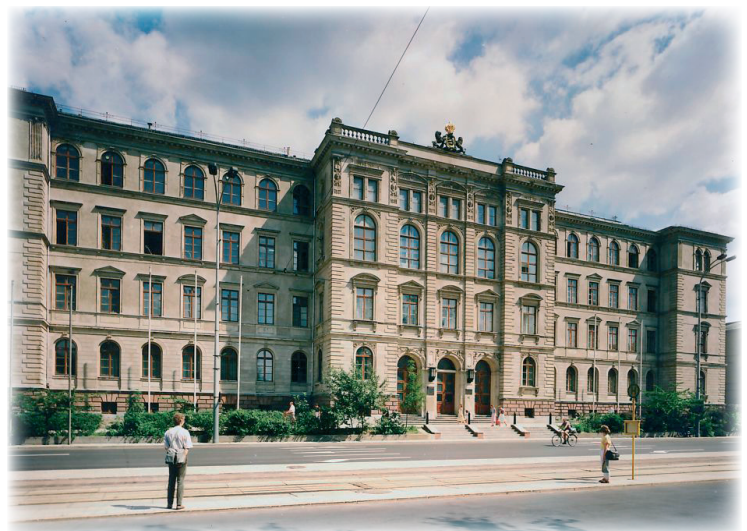
Figure: Behind the historic facade of the Technical University (TU) Chemnitz there is a state of the art IP infrastructure. Source: TU Chemnitz
